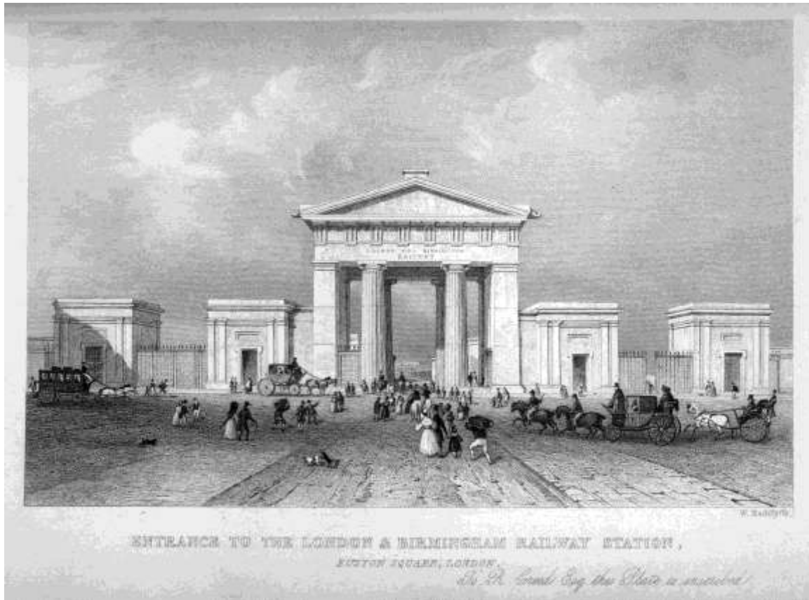
Entrance to Euston Station (now demolished). © British Library Board (074019).
