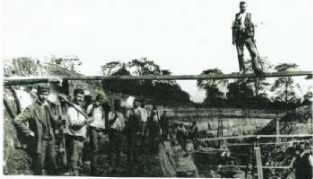
About 1910. This picture shows a large gang of men working in one of the quarries removing the overburden. There are a lot of trestles and planks bridging the quarry to provide access to the dump side where the overburden spoil was tipped from the barrows.
