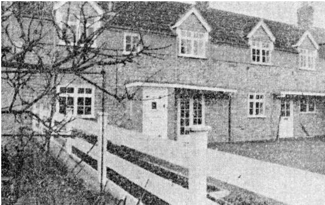
House in Carlow Street said by Wilfred Roberts to be where Benjamin and his family lived. His workshop was at the back (house much altered) Chronicle & Echo 1975
